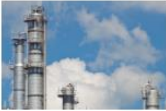
Air Treatment & Odor Control
